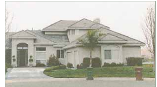
^ Modulation in building mass has been applied here effectively to reduce the visual impact of a large house.
